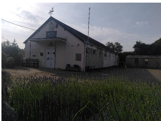
Recreation Hall, Long Hanborough
